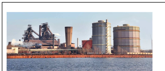
Figure 14 A steel plant in europe that emits 3,000,000 MT of CO 2 /yr.
